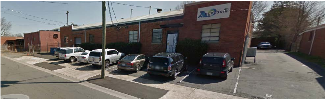
Properties to the north are developed with industrial uses.
