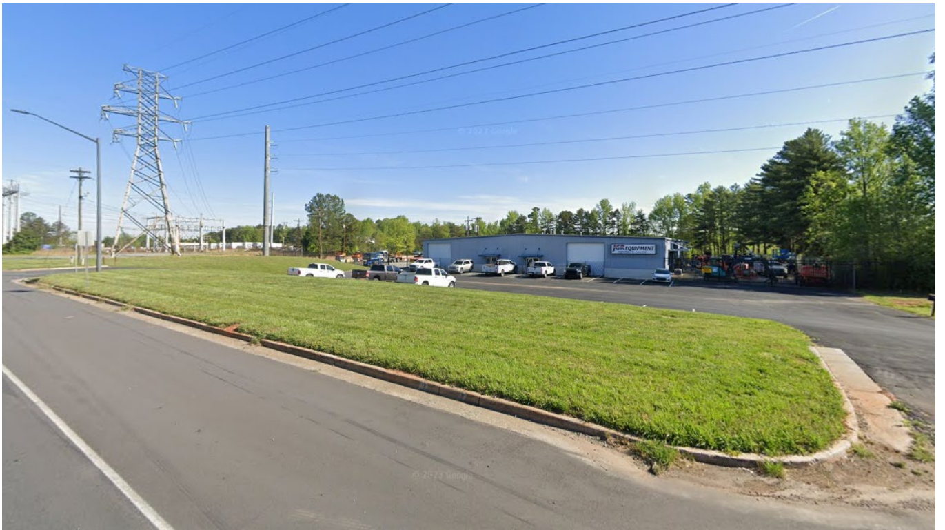
View of an equipment rental facility located to the northeast of the site across Brookshire Blvd.
