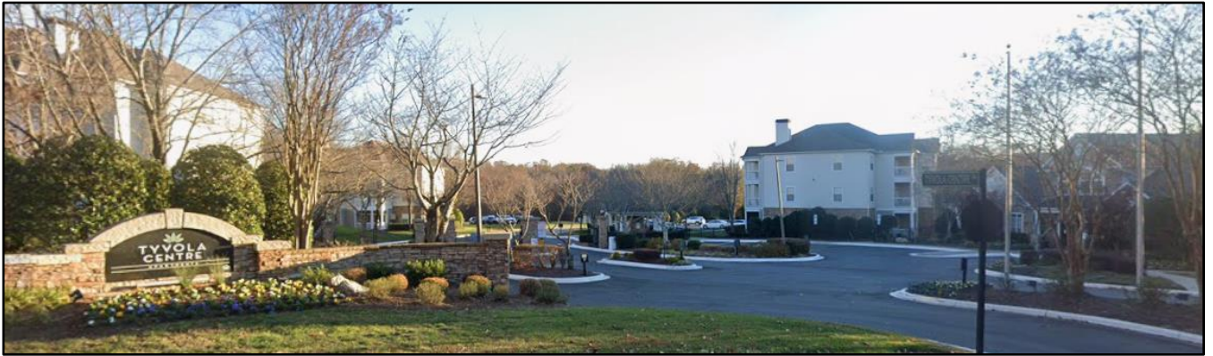
View of garden-style multi-family apartment development located across West Tyvola Road from the site, typical of the development pattern along West Tyvola Road.
