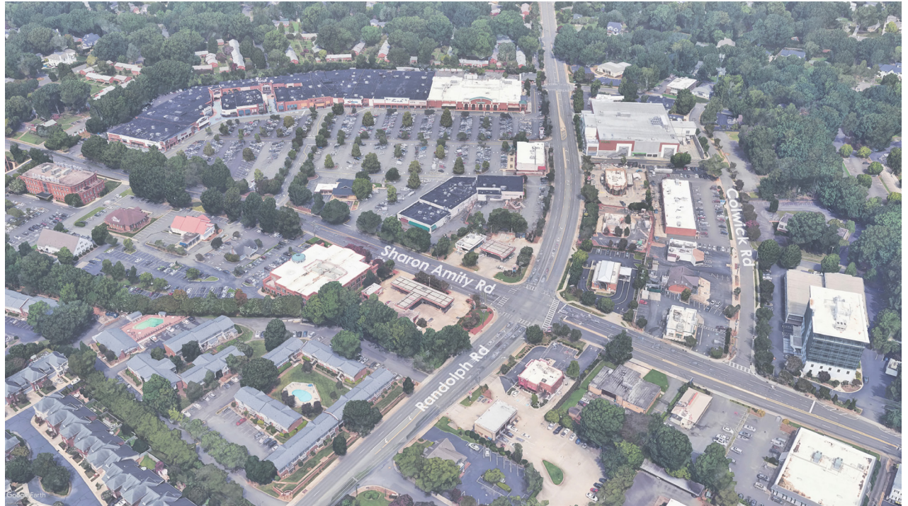
FIGURE 8: AERIAL OF EXISTING CONDITIONS
