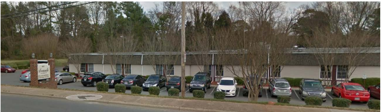
Curis Transitional and Rehabilitation Center abuts the property to the south.
