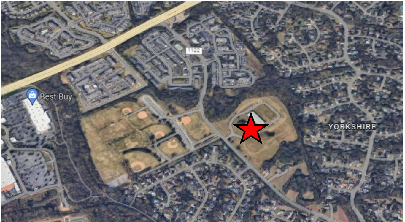
The site, marked by a red star, is surrounded by a mix of uses including single family residential, multifamily residential, and recreational uses.
