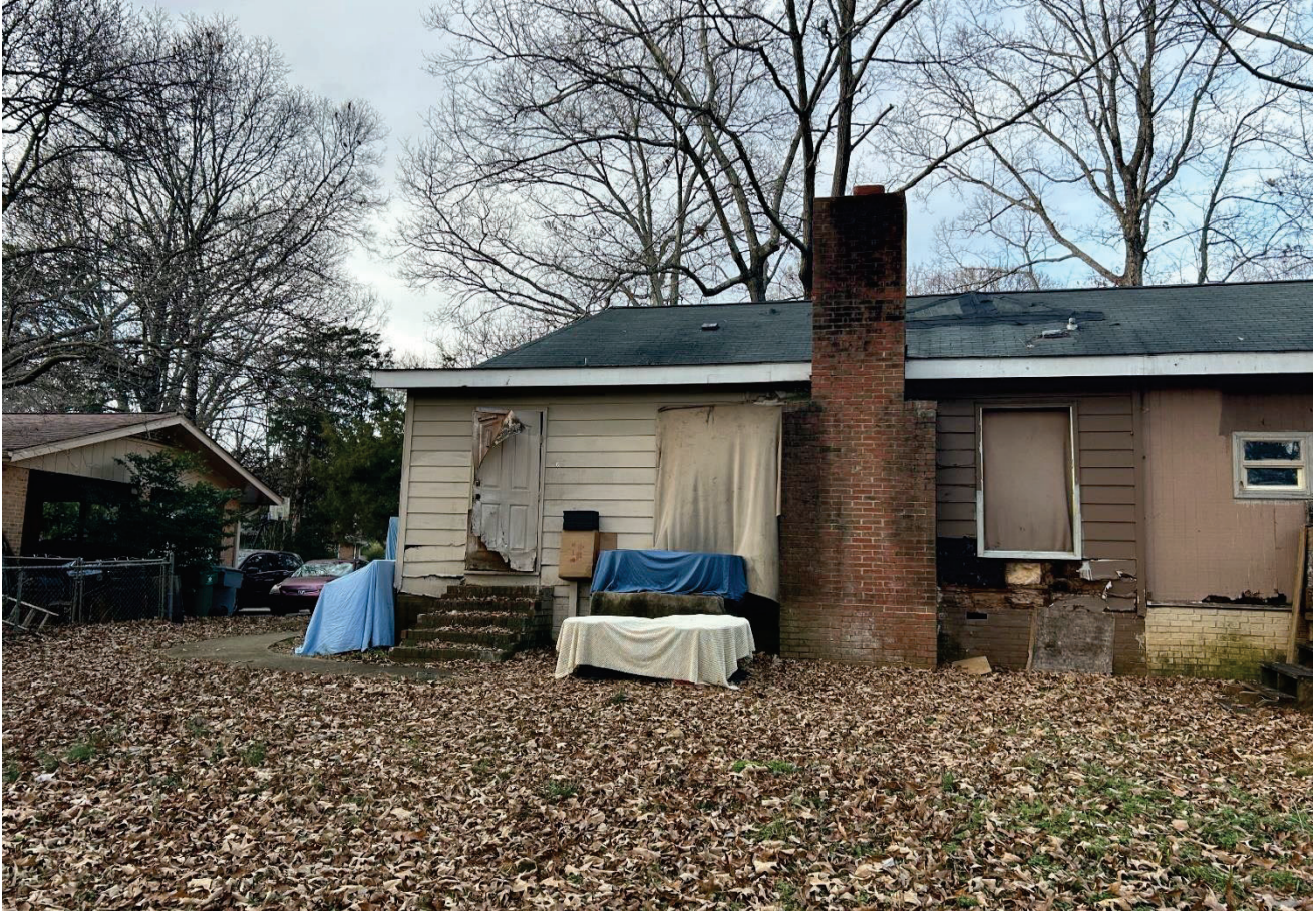
Rear of structure
