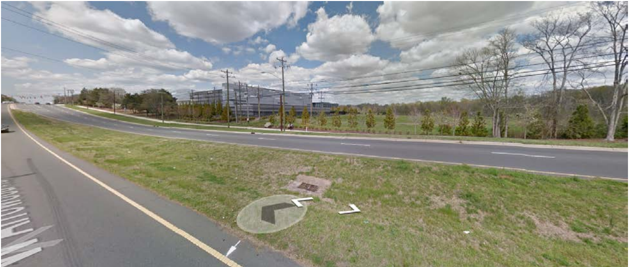
North of the site, across West Arrowood Road is the offices and server farm at Spectrum's campus.
