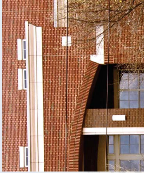
Simplified pilasters, piers, and banding
