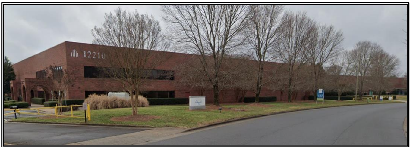
The property to the west along Vance Davis Drive is an office and distribution center.
