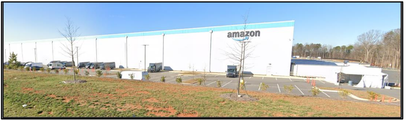
The property to the south along Old Statesville Road is the Amazon distribution center.
