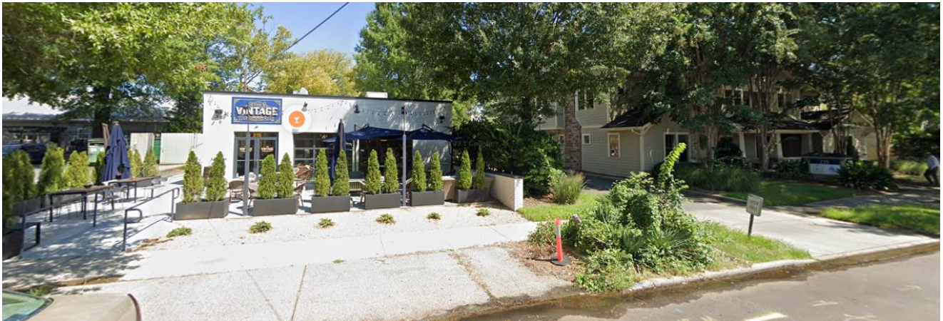
View of adaptively reused buildings north of the site along East Worthington Avenue. Many of the surrounding properties were once single family homes, warehouses, or auto-oriented commercial uses that have since been revitalized into restaurants, retail spaces, and offices.
