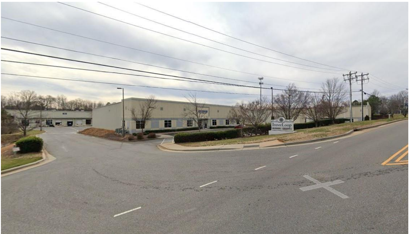
View of warehouse/industrial properties west of site on the south side of David Cox Road.
