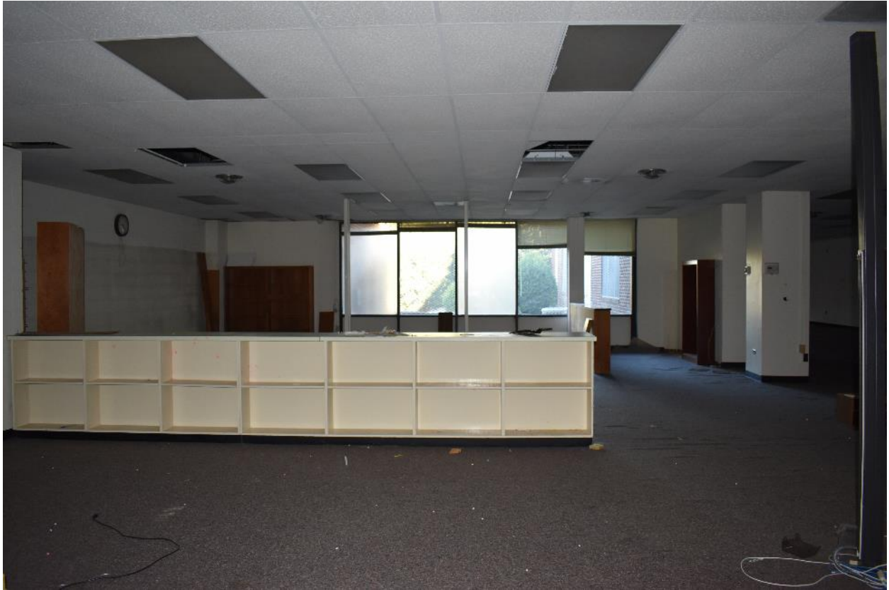
1970 library looking west.
