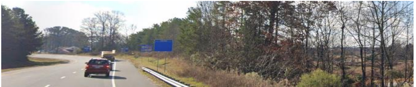
Street view of the Interstate 485 ramp to the north of the site. Provide caption for Street view (use north of site).
