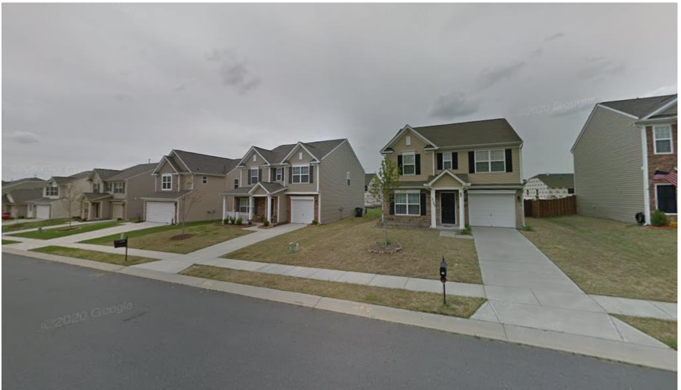
View of houses along Verde Creek Road in a single-family subdivision located to the northeast of the site.
