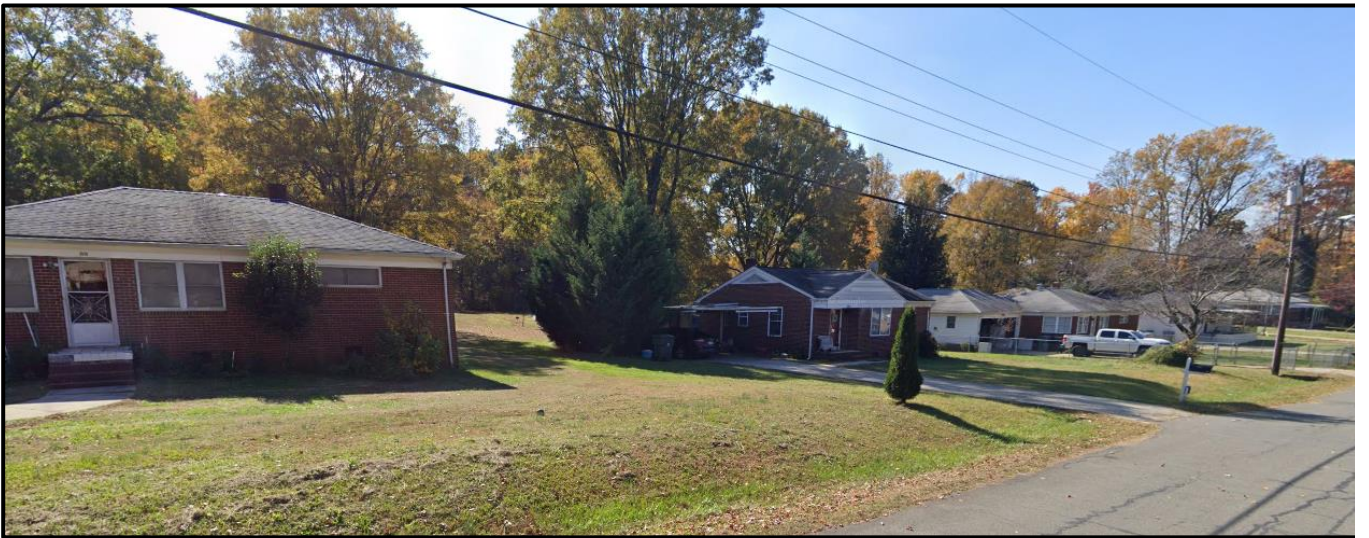
The property to the north along Juniper Drive is developed with single family homes.
