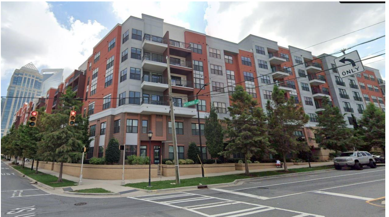
View of an apartment building located west of the site at the corner of West Morehead and Winnifred Streets.
