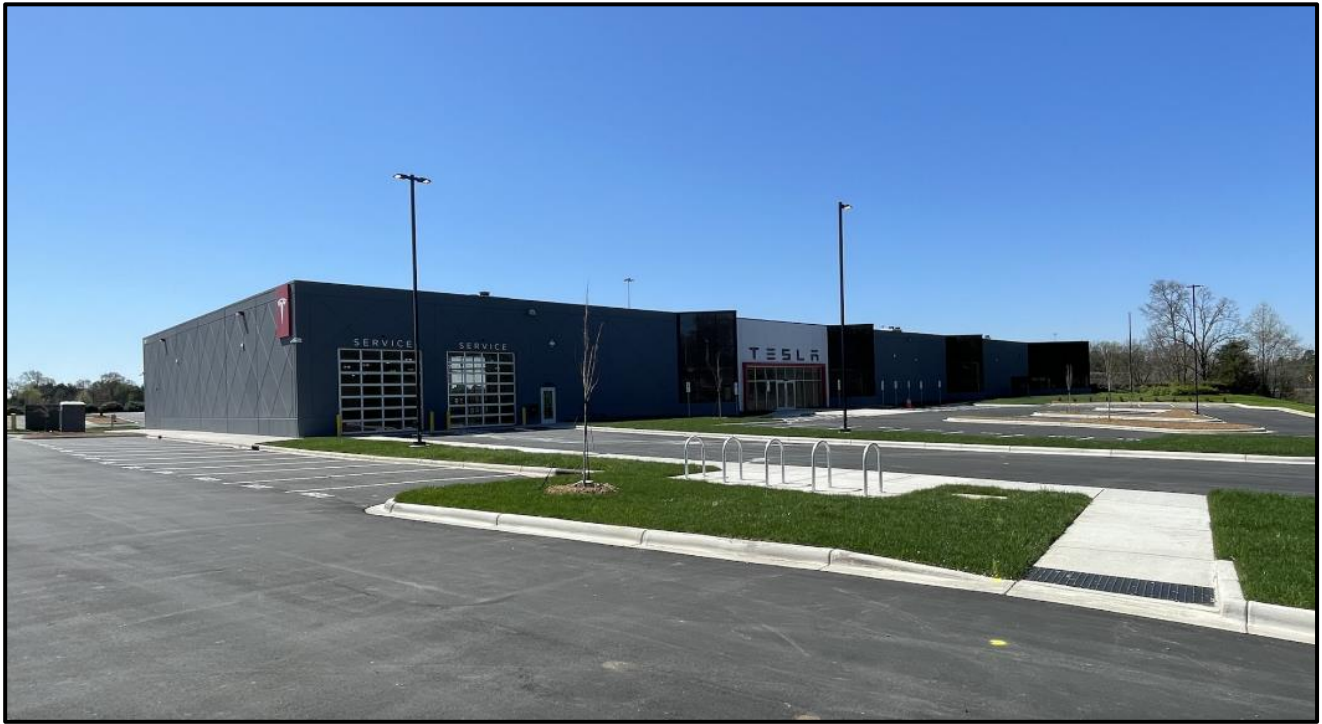
The property to the south along Twin Lakes Parkway is developed with a Tesla auto dealership.
