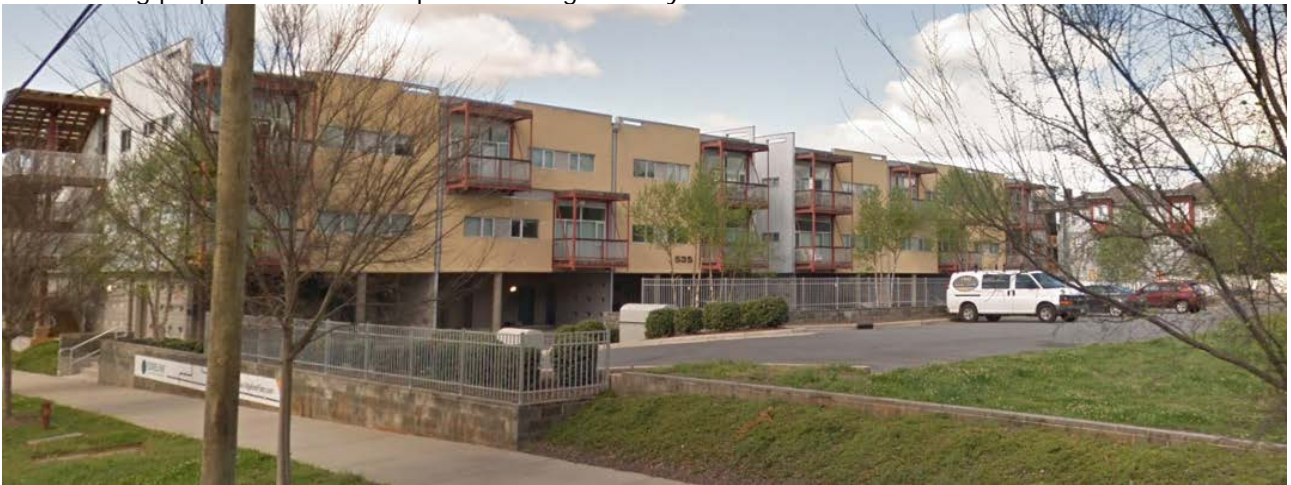
Multi-family dwellings are located near by.
