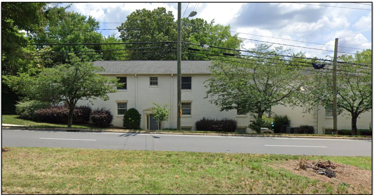
East of the site are multi-family dwellings.
