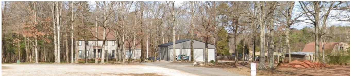
Street view of contractor office with outdoor storage illegally operating on the site as seen from Shopton Road West.
