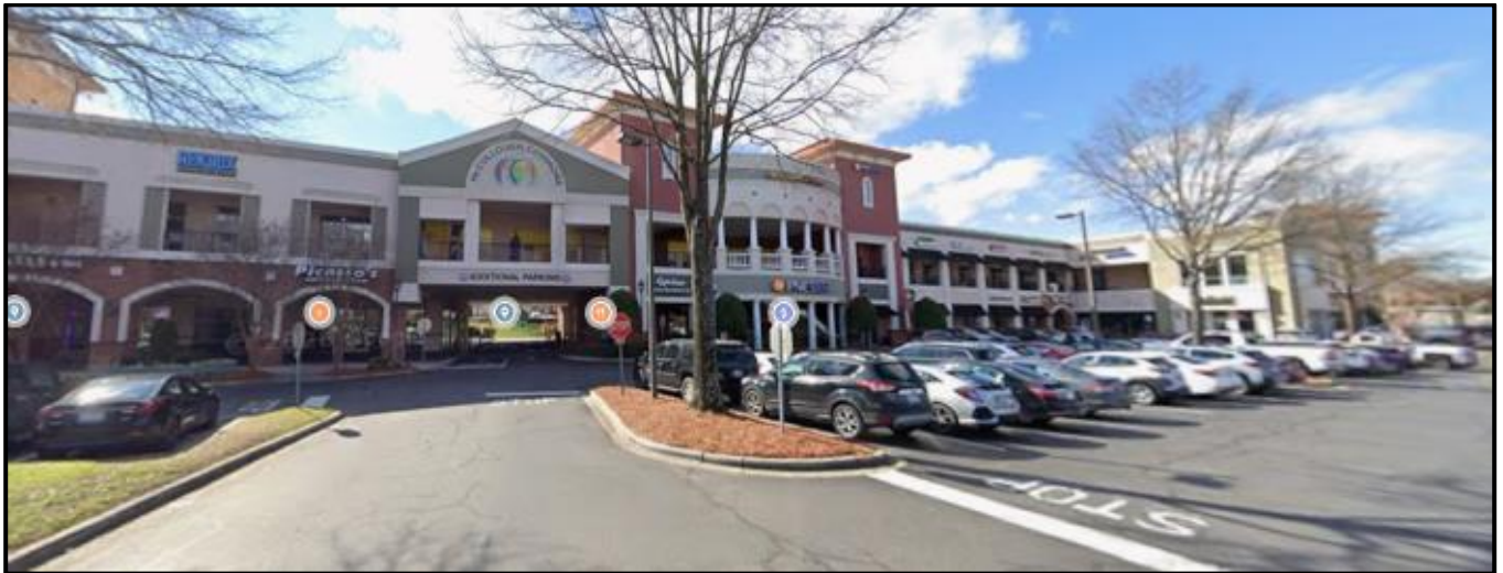
The property to the south along East WT Harris Boulevard is developed with retail shops.
