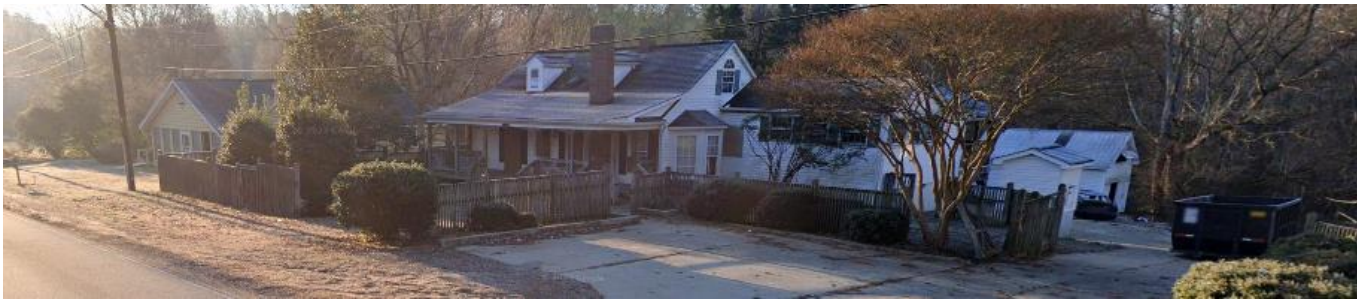
Street view of single family residential uses to the east of the along Mount Holly Road.
