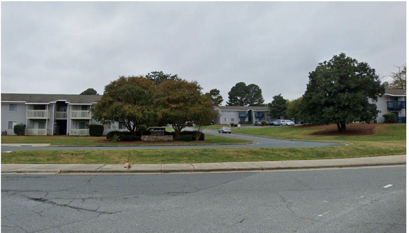
View of the Meadowbrook Apartments entrance located southwest of the site at the corner of Grier Road and Newell-Hickory Grove Road. One of the two apartment developments to the south of the site.
