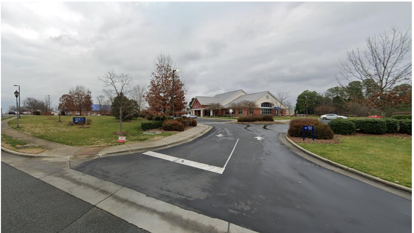
View of the financial institution occupying the northern portion of the parcel shared by the proposed site.
