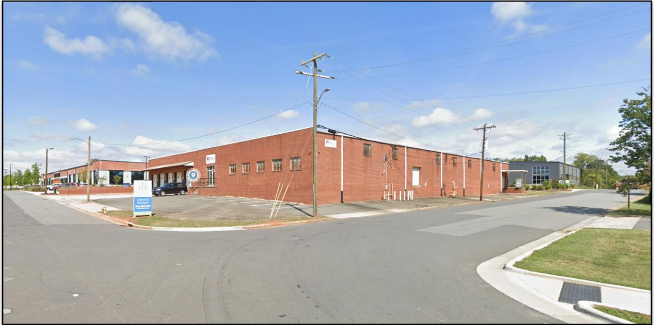
The site Street view on Jay Street has an existing structure.
