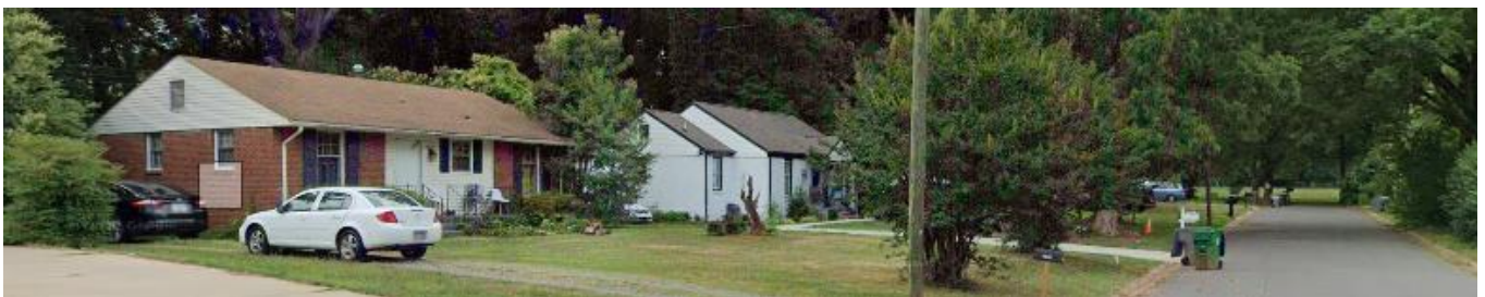
Streetview of single family detached dwellings to the east and south of the site along Grapevine Drive.
