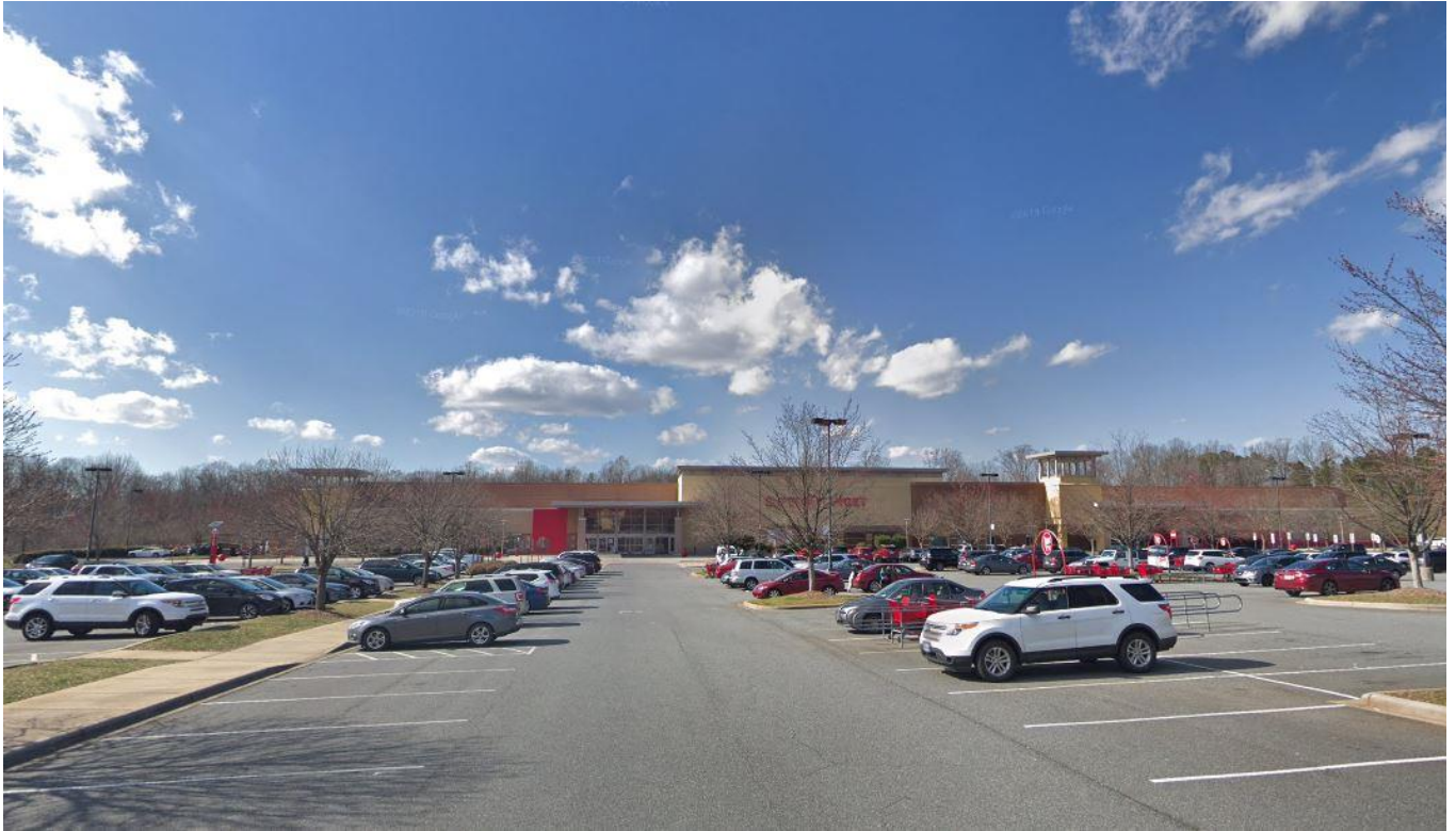
View of the Super Target located to the north across West WT Harris Boulevard. Retail is the predominate land use in this area.
