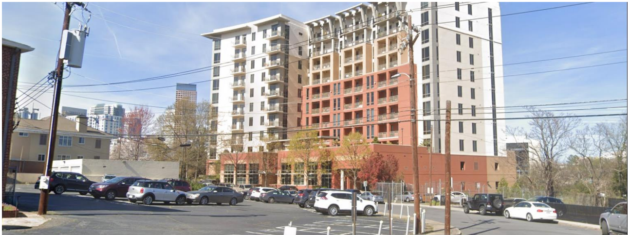
On the opposite side of Royal Court are condominiums.
