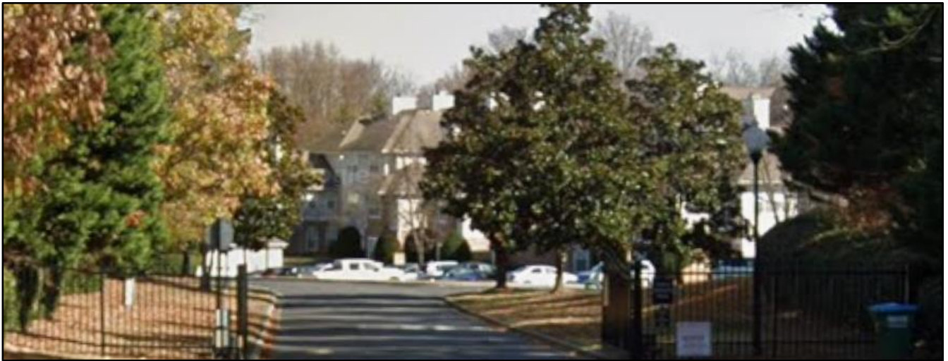
View of a multi-family apartment development looking northeast from Sandy Porter Road. The multi-family development is abutting the subject site to the northeast and is designated as the Community Activity Center Place Type by the 2040 Policy Map .
