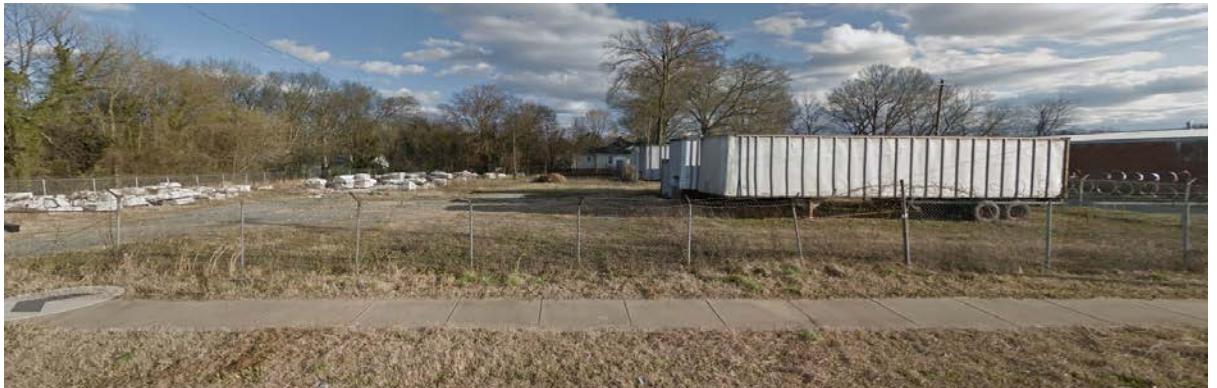
The subject property is zoned I-2 (general industrial) and undeveloped.
