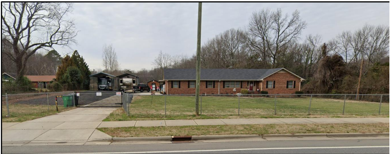
The property to the south along Statesville Road is developed with large lot single family homes.
