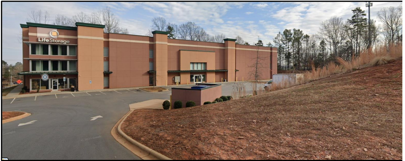
The property to the north along Legranger road is developed with a storage facility and a Duke Energy substation.
