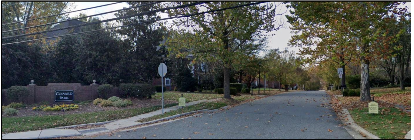
The property to the west along Mallard Creek Road is developed with single family homes.
