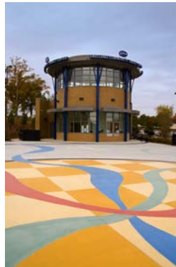
Eastland Transit Facility opens
