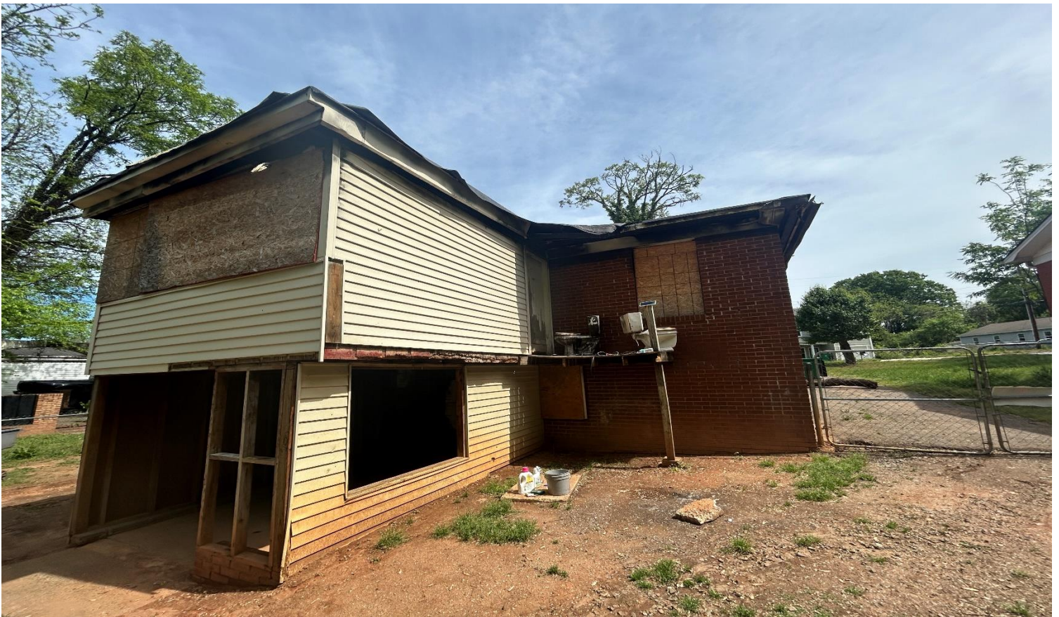
Rear of structure
