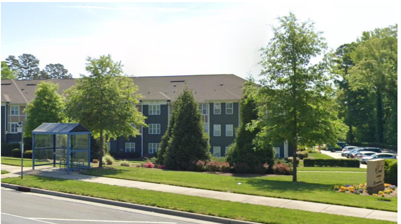
View of a retirement facility located west of the site along Mt. Holly-Huntersville Rd.
