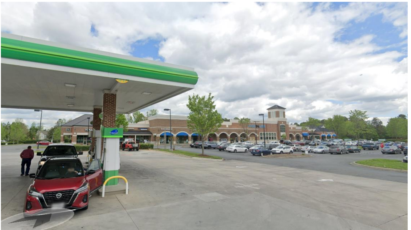
View of a shopping center development located approximately ¼-mile northwest of the site across Mt. Holly-Huntersville Rd zoned B-1(CD).
