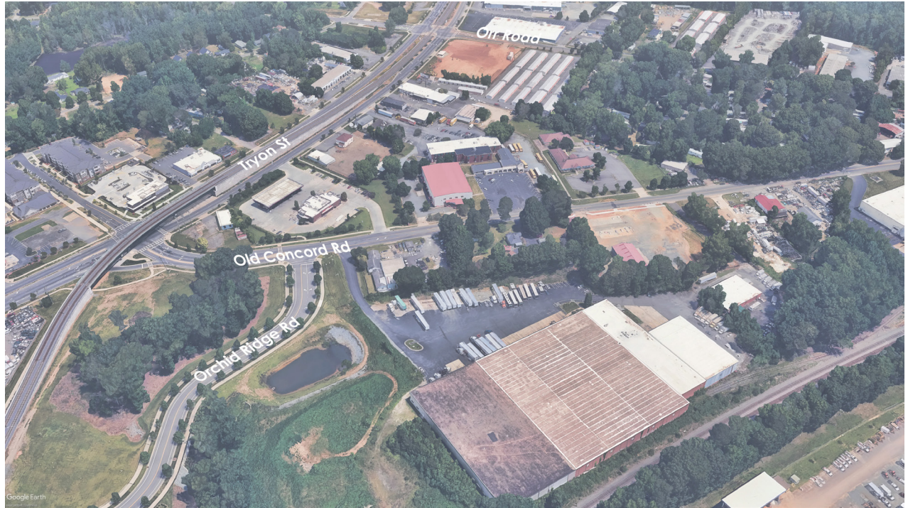
FIGURE 11: AERIAL OF EXISTING CONDITIONS
