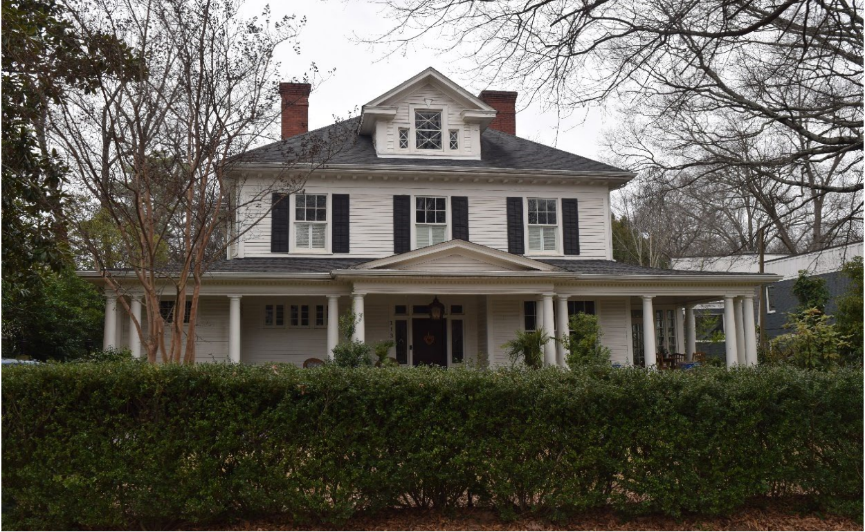
Front of house (east elevation), view west
