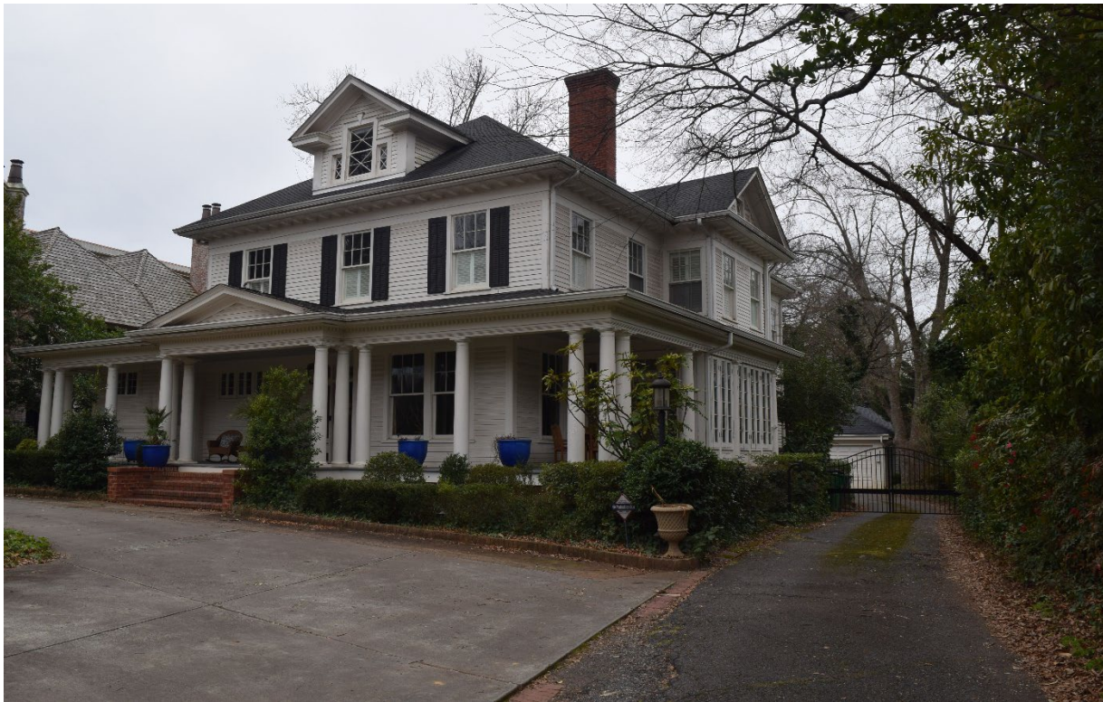
Northeast corner of house, view southeast.
