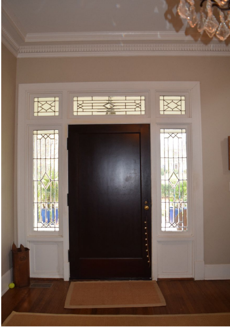
Front door detail, view east
