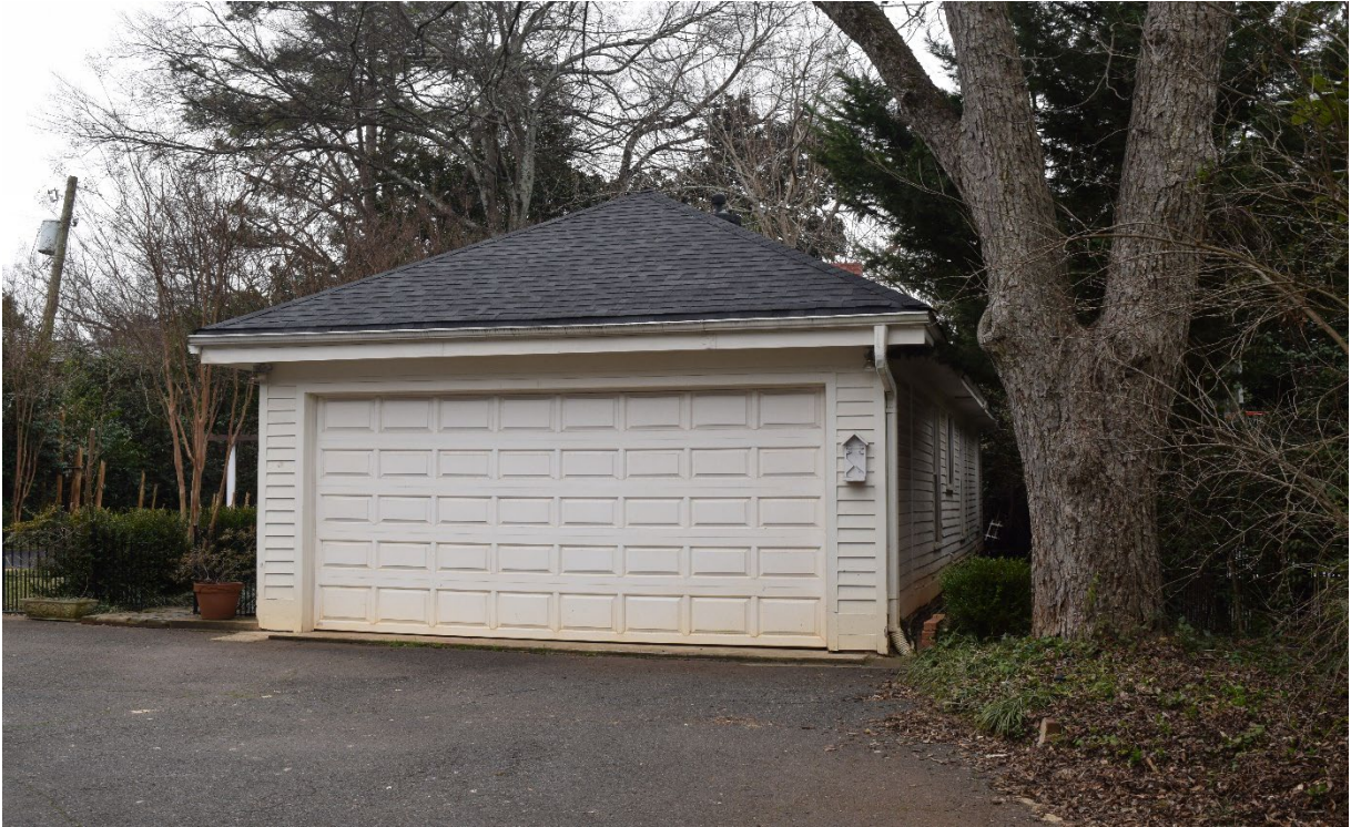
East elevation, servant's quarters/guest house, view west.
