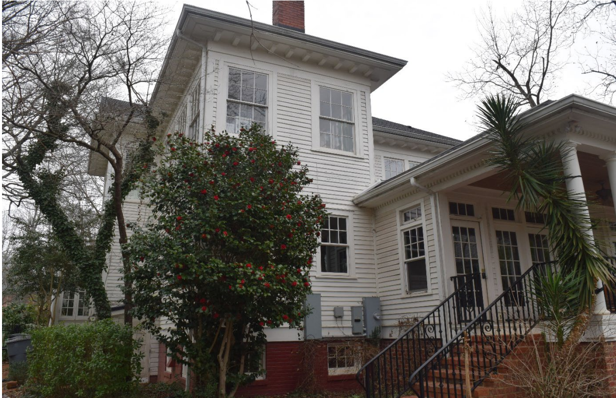
Northwest corner of house, view southeast.
