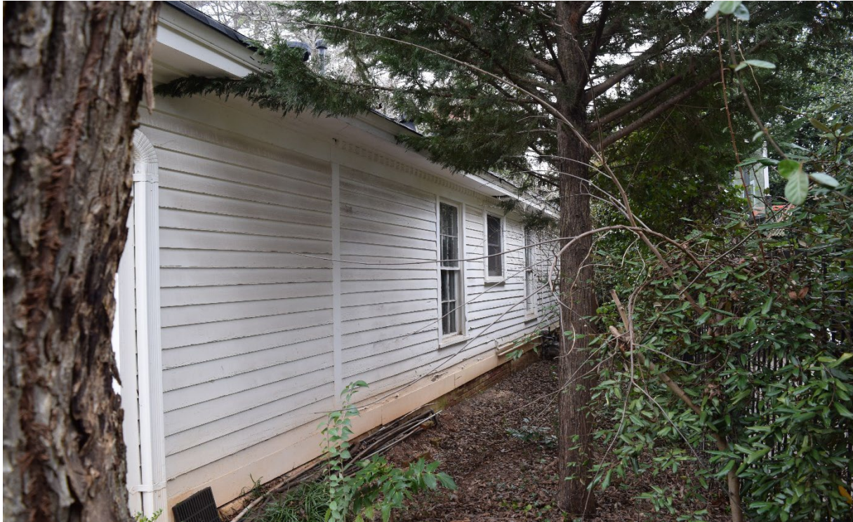
North elevation, servant's quarters/guest house, view southwest.
