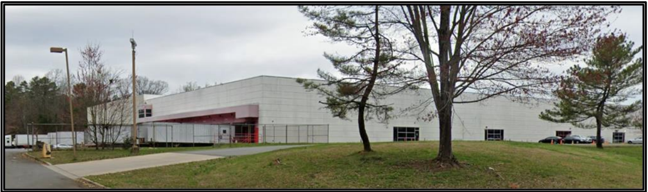
The property to the south along Morris Estate Drive is developed with a warehouse use.
