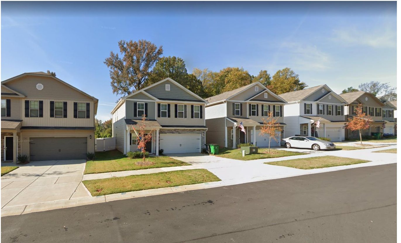
South of the site is a neighborhood of single-family residential homes.
