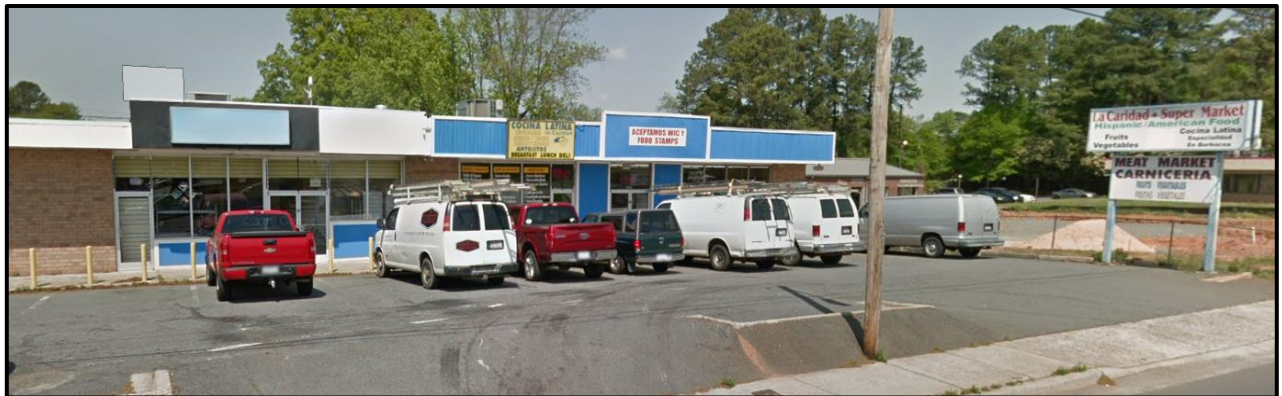
The property to the south along North Sharon Amity Road is developed with retail uses.
