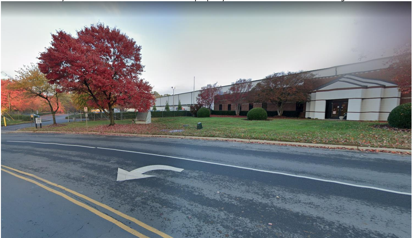
To the north of the site there is a warehouse/distribution center.
