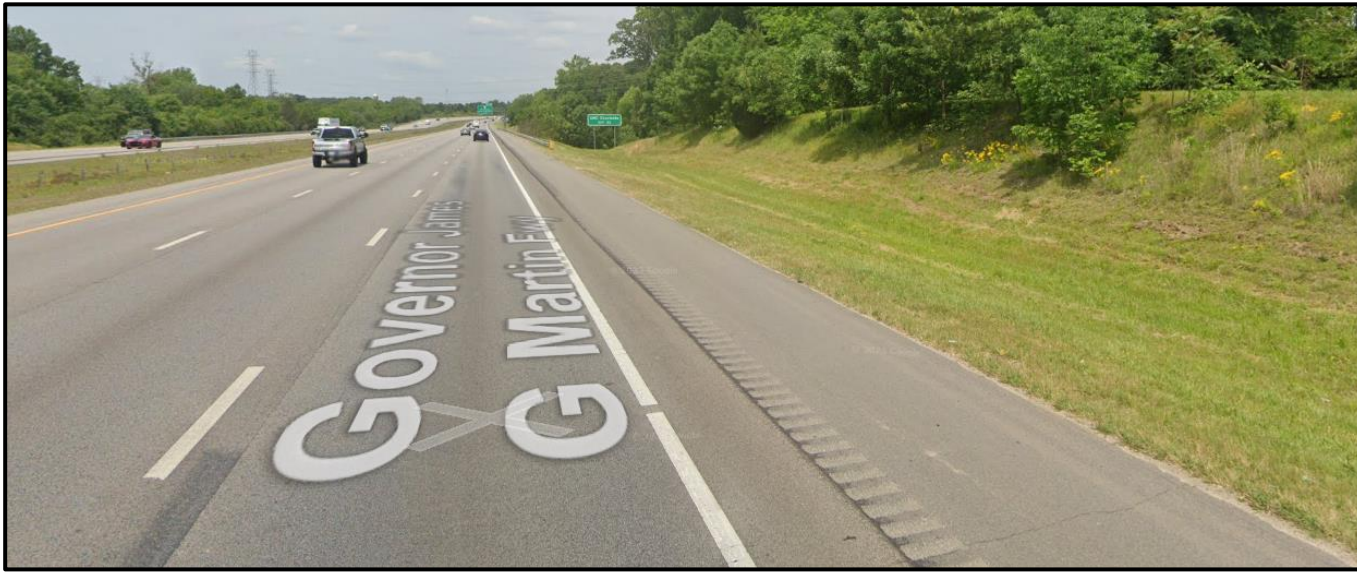
Interstate 485 is to the south of the property.
