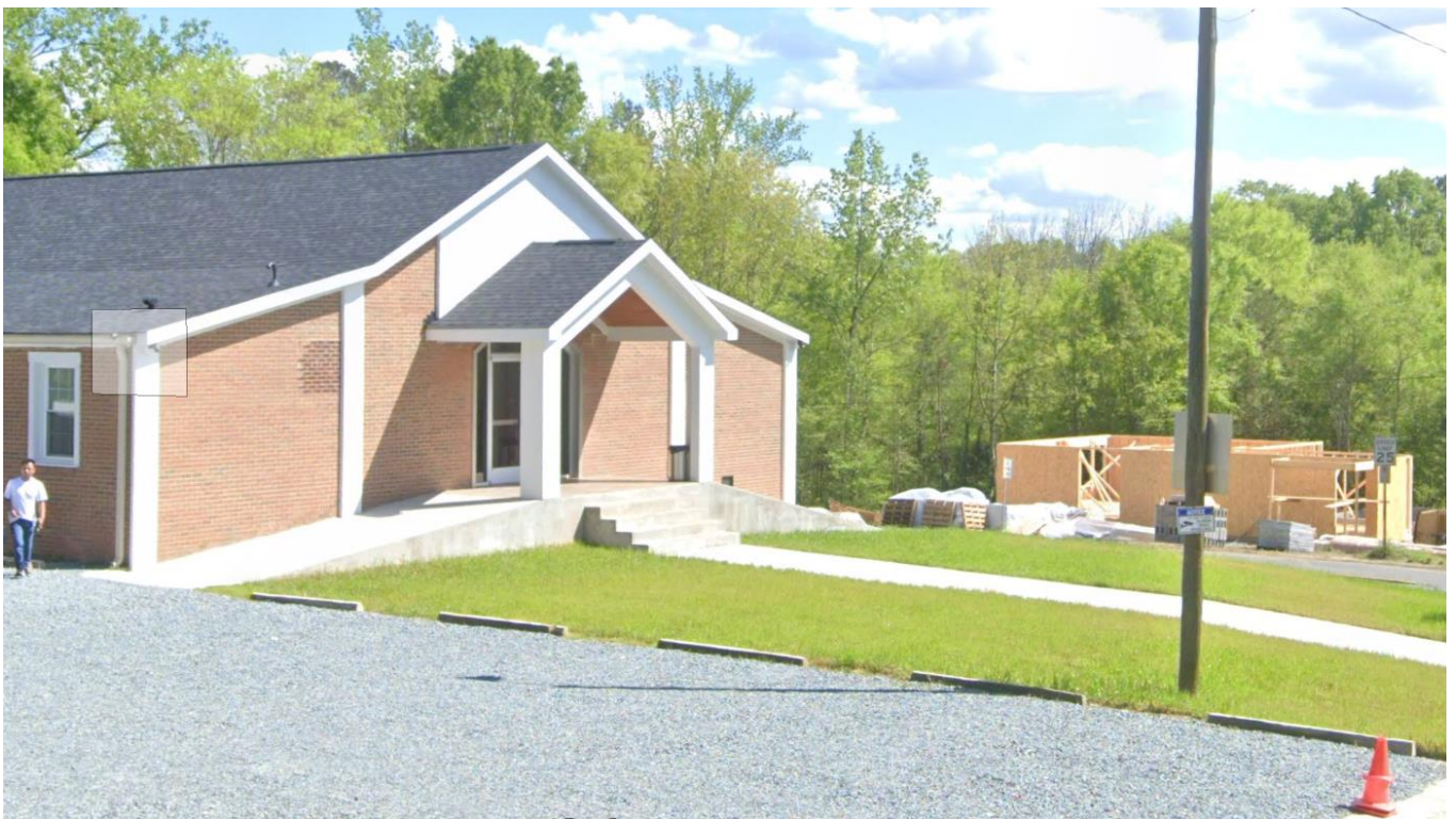
View of a church and new single-family house located southeast of the site along Pawley Dr.
