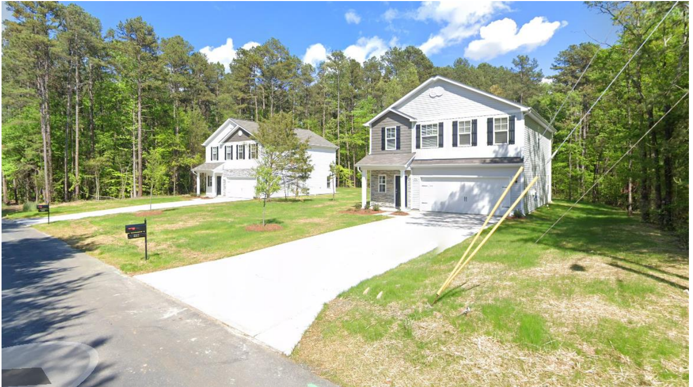
View of single-family houses located on Pawley Dr. southeast of the site.
