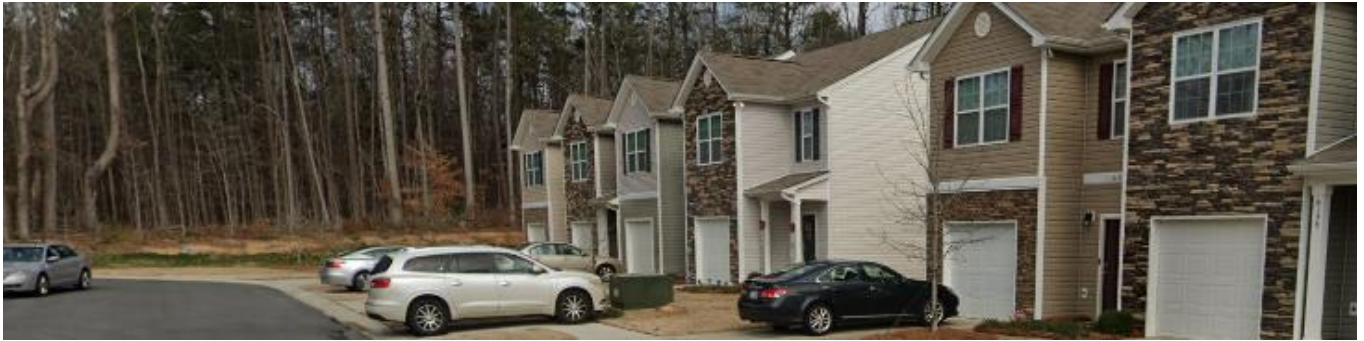
Street view of multi-family attached residential use to the south of the site along Guildford Hill Lane.
