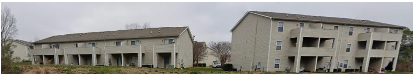
Street view of multi-family residential use to the north of the site across Cagle Avenue.
