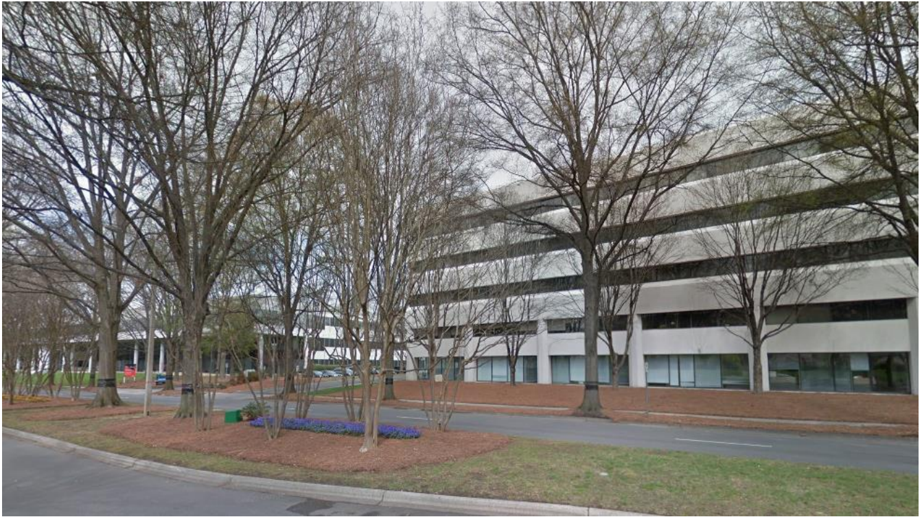
View of the site looking north from Rexford Road. The site is developed with two office buildings.
