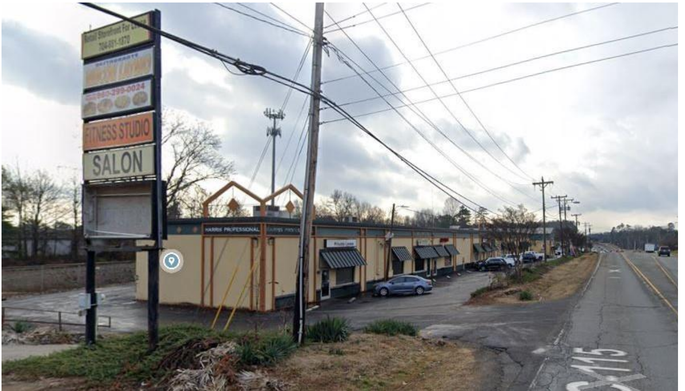
View of retail uses along the west side of Old Statesville Road.
