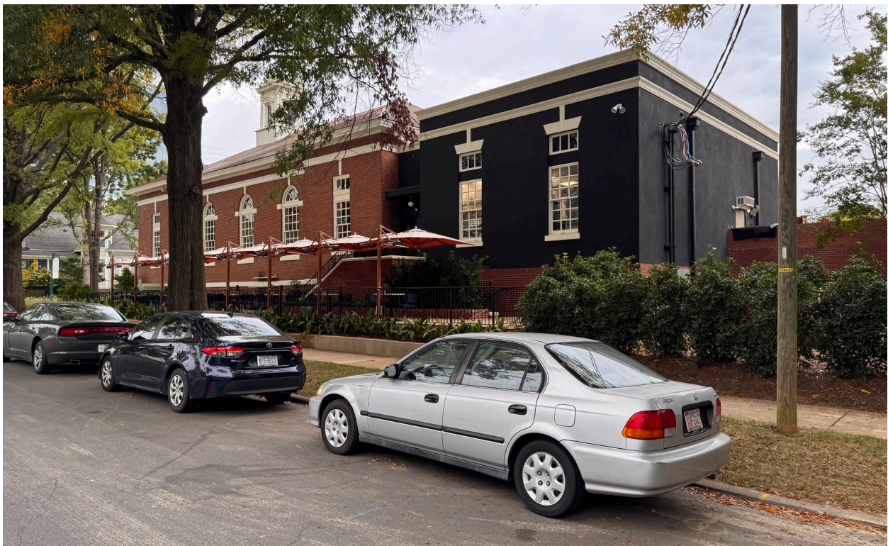
8. Looking north, the southwest elevation from East Worthington Avenue.
