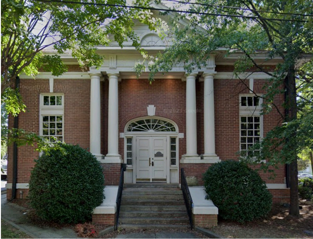
12. View of front facade in 2022.
