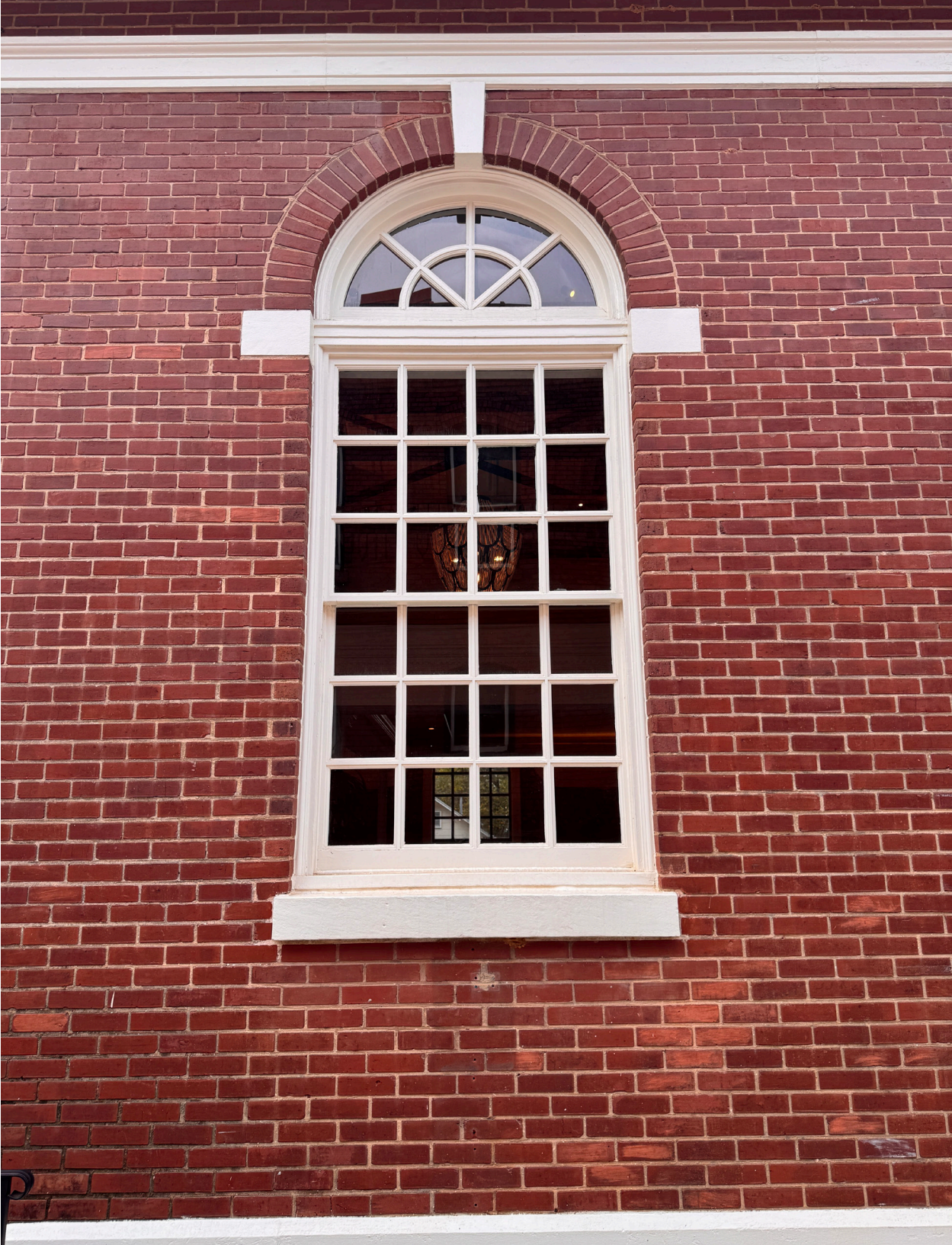
9. View of typical exterior window.
