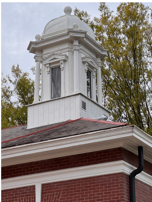
Figure 10. Current photograph of cupola.
