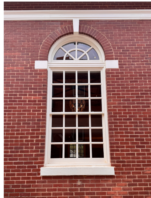
Figure 9. Current photograph of building window and belt coursing.
