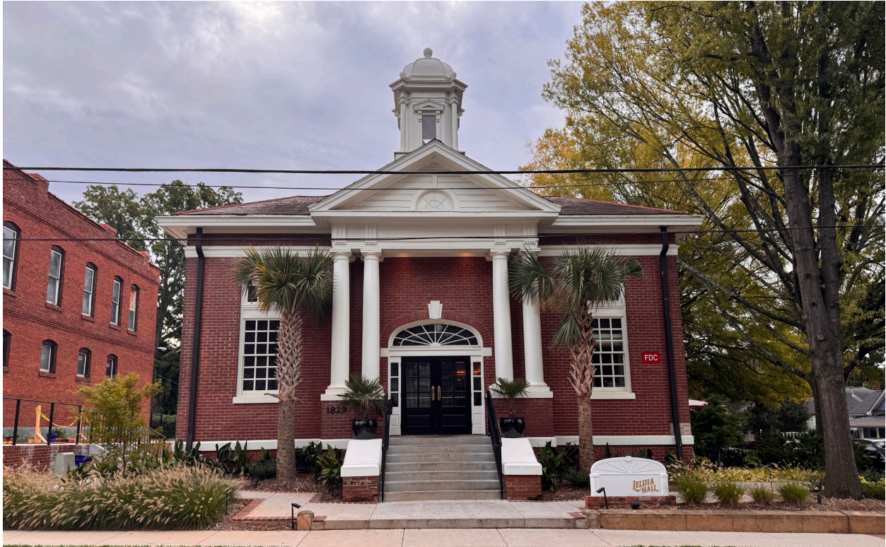
1. Looking southeast, the front northwest facade of the building.
