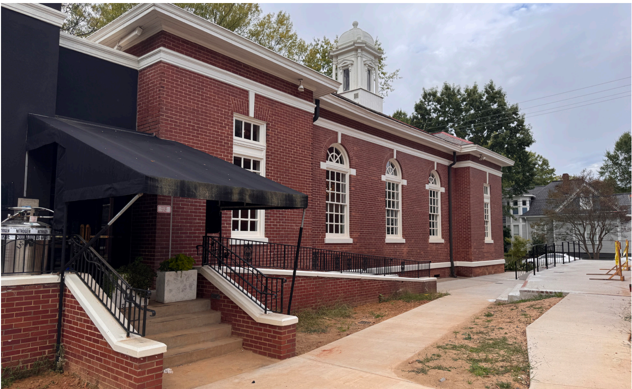
4. Looking northwest, view of the northeast elevation.
