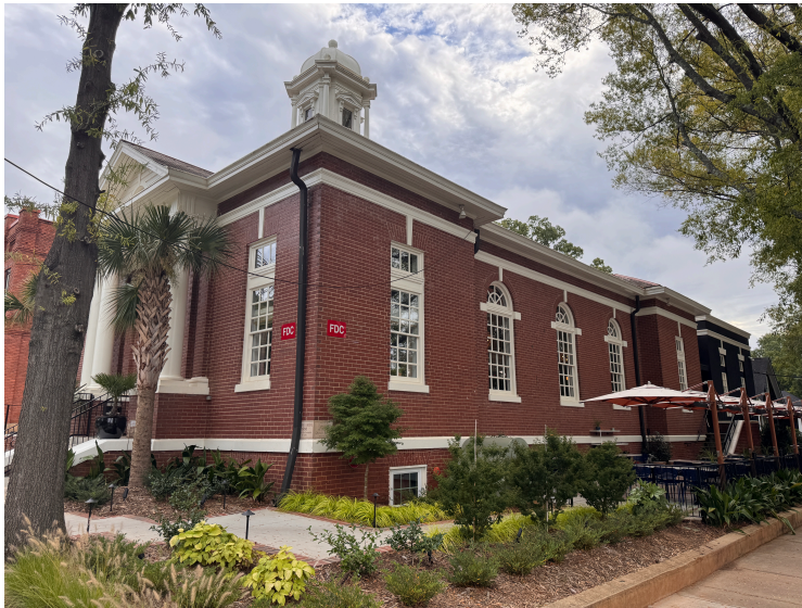
Figure 8. Current photograph of the southwest elevation.
