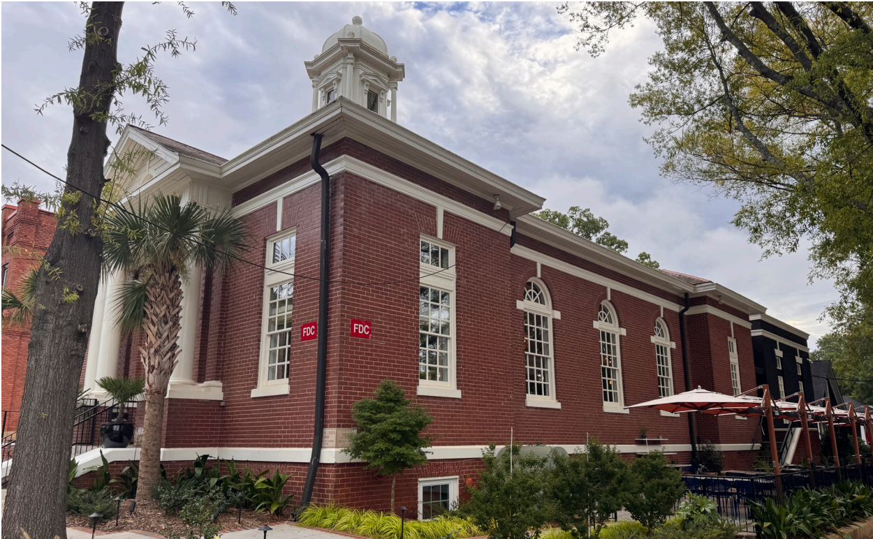
6. Looking northeast, the southwest corner of the building.
