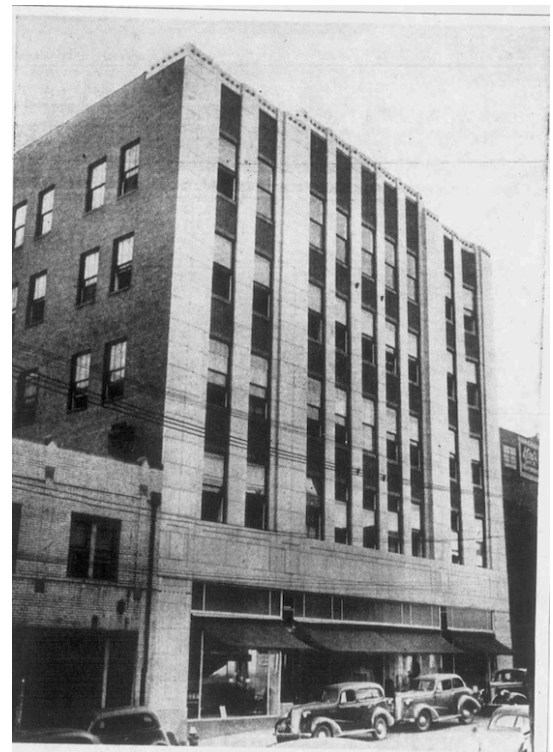
Figure 5. 1938 photograph of the Belk Brothers building addition facing East Fifth Street.
