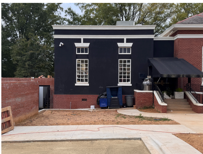
Figure11. Current photograph of the ca. 1999 rear addition.
