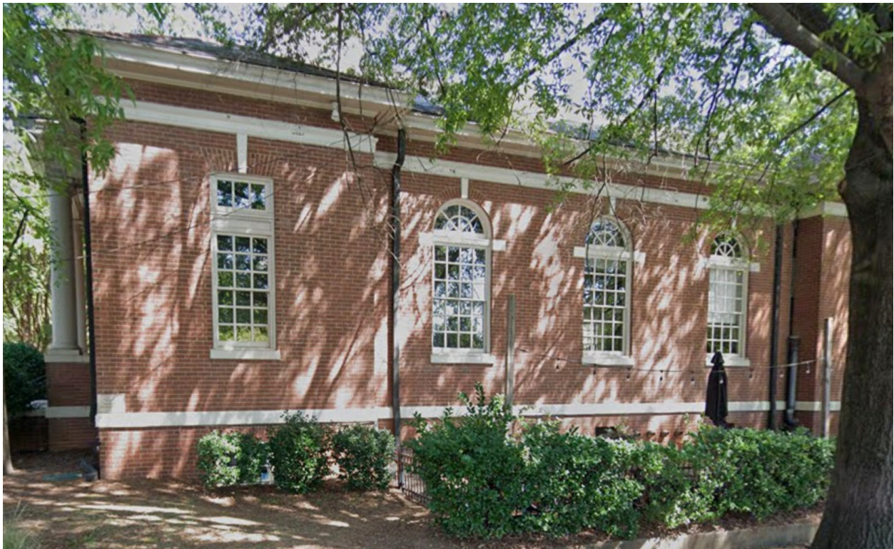
15. View of southwest elevation in 2022.
