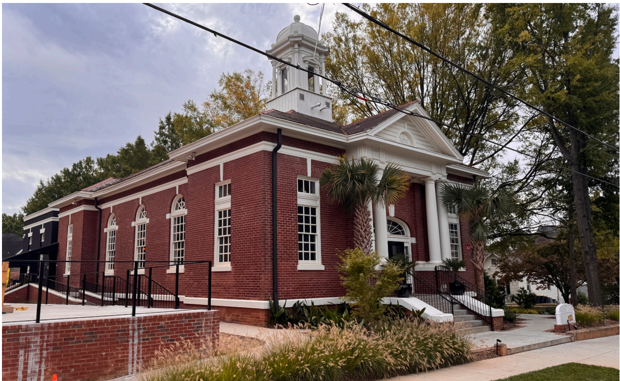
2. Looking south, the north corner of the building and the northwest and northeast elevations.
