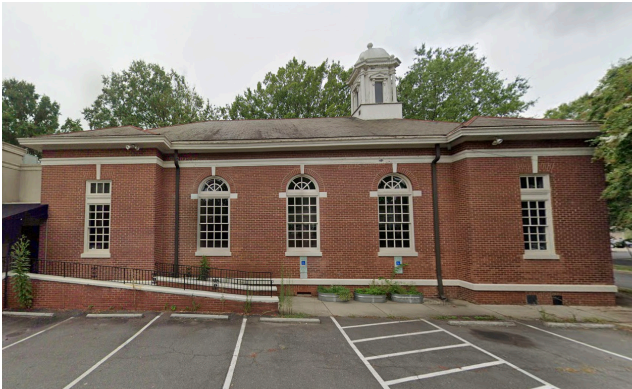
13. View of northeast elevation in 2022.
