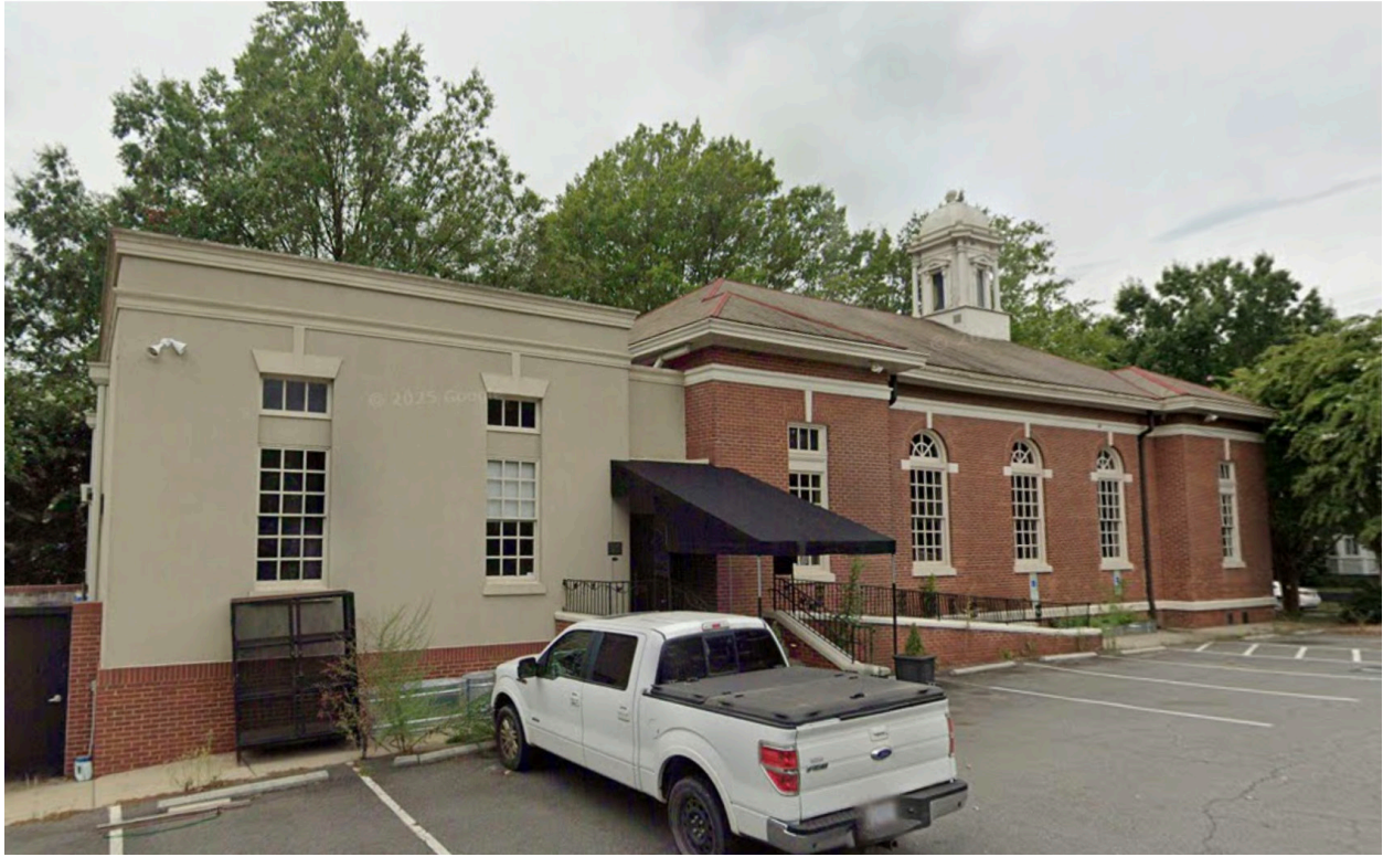
14. Additional view of northeast elevation in 2022.
