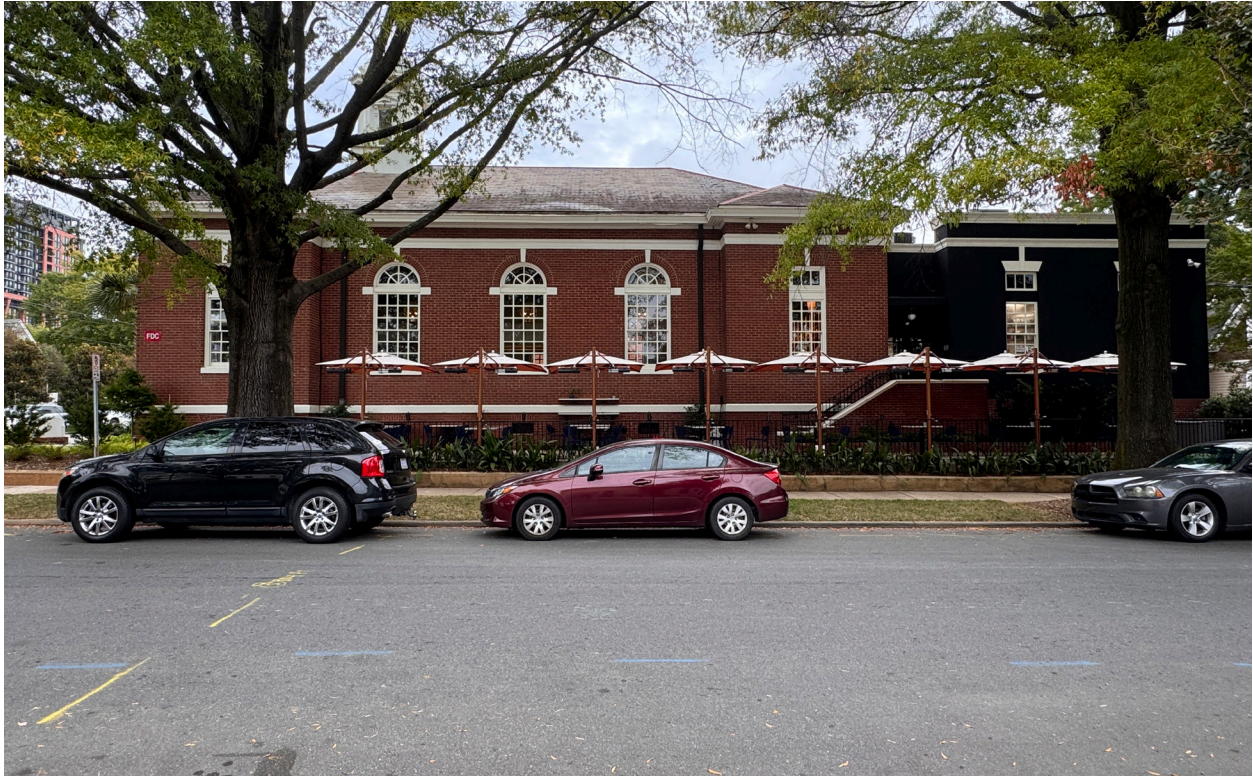
7. Looking northeast, the southwest elevation of the building.
