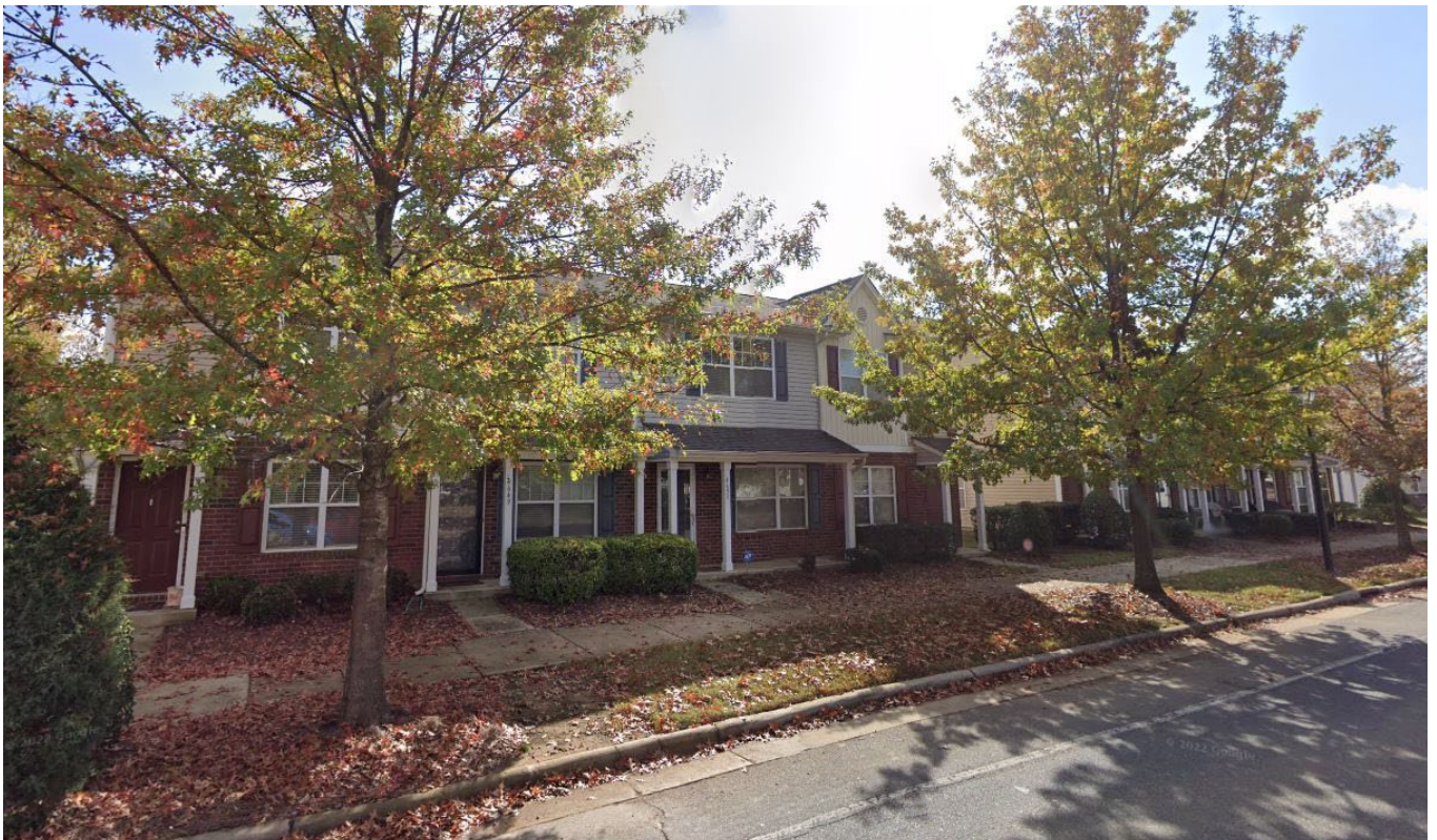
View of the townhome development located along Johnston Oehler Road southwest of the site.
