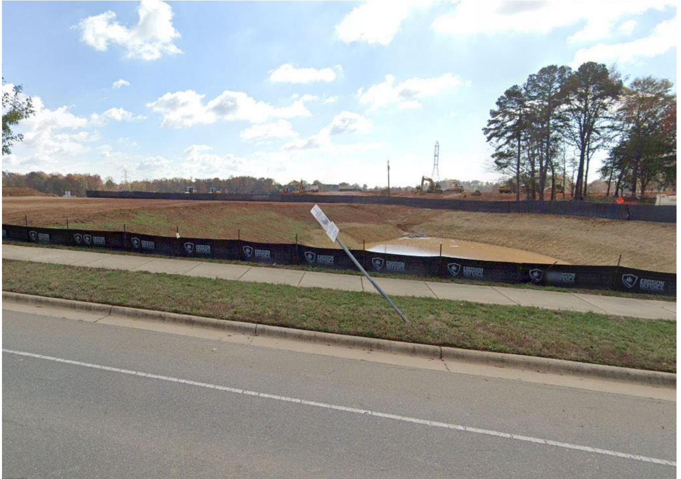
View of the multi-family development, currently under construction, located on Johnston Oehler Road southeast of the site.
