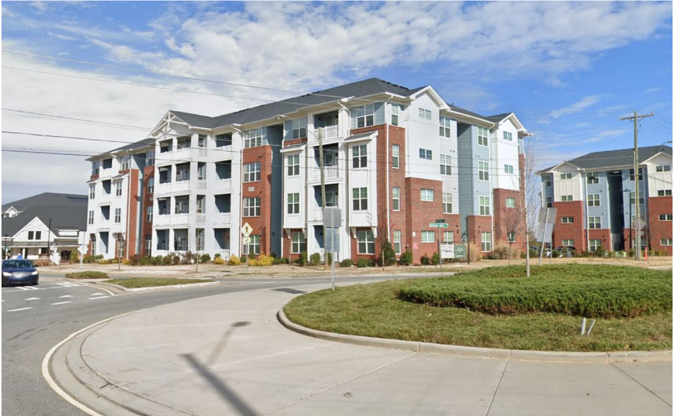
View of the multi-family development located at the corner of Prosperity Ridge Road at Johnston Oehler Road west of the site.
